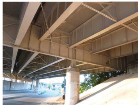
UNIT I - PIN REHABILITATION
