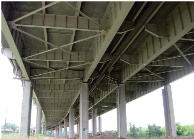
UNIT 3 PIER GRDR 13 REHABILITATION WORK AREA
