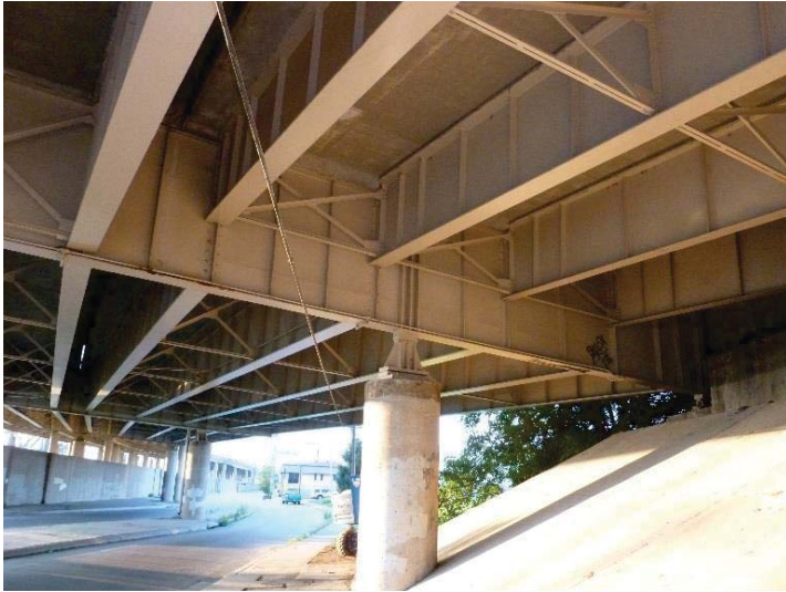
UNIT 1 PIN REHABILITATION WORK AREA
