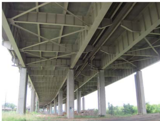
UNIT III - PIER GIRDER 13
