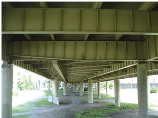
SPAN 31, UNIT III WB – GIRDER 3
